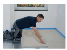
Press the element firmly down along the rebate. Some of the adhesive will be forced out of the joint.
