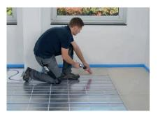
Start with the remainder piece ( $\ge 20$  cm) so that you lay in subway bond (joint offset  $\ge 20$  cm). Apply two adhesive strings to the rebate (ø approx. 5 mm).
