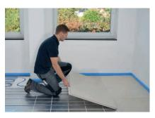
Place element onto the rebate, push it into the correct position. Skin formation time of the adhesive: approx. 4 min. Rebates have to be adehred during this time.
