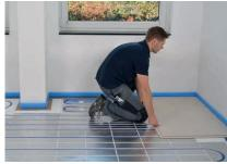
Start laying in the left-hand corner of the room. Do not press the edge insulating strips together as you do so.
