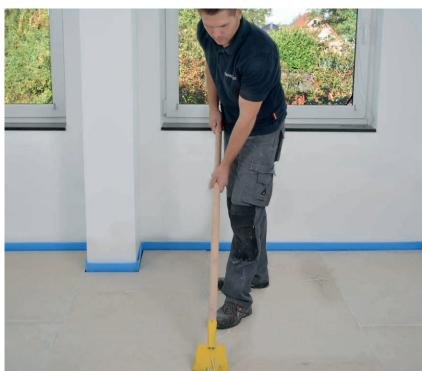
After a 24-hour drying period, the excess adhesive can be removed with a spatula. After that, the floor covering can be laid (Notice our material releases  $\rightarrow$  Datasheets floor covering | adhesive).
