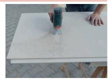
Shorten the last element in a row to length (e.g. using a circular saw blade Diamaster or a jigsaw blade T141 HM, Bosch).
