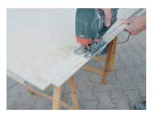
To start laying, saw off the projecting fold of the first element and do the same for the complete first row.
