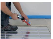
Apply the first adhesive string close to the inside edge, and the second one in the last third of the rebate (approx. 5 m<sup>2</sup>/cartridge).
