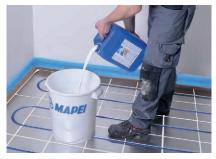
Mix a canister of Latex Plus and a bag of Planitex D10 (~ 11 m<sup>2</sup>) using a slow-running mixer (max. 400 rpm).
