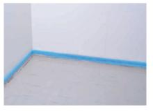
Allow to dry at 20 °C room temperature for at least six hours – cooler temperatures (min.  $10^{\circ}$ C) extend the drying period.
