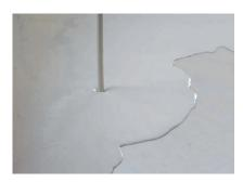
Add the load-bearing layer manually or using a screed pump and seamlessly distribute onto the completely dry contact layer.
