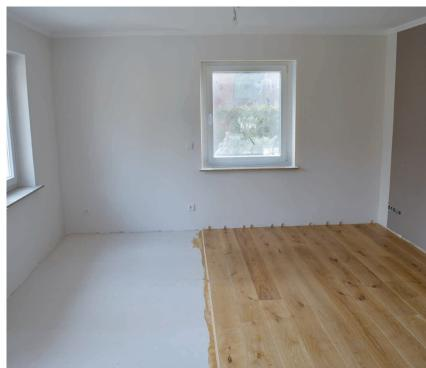
At the earliest after a four-day drying period, perform the heating protocol CompactFloor LIQUID. Subsequently, after the control of the residual moisture, the floor covering can be laid.
