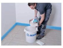
For the load-bearing layer, mix one bag of Planitex D10 with 6.5 I water and add one bag of fibres (250 g).
