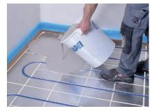
Subsequently, pour the mixture onto the dust-free and clean heating elements.
