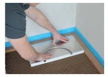
First adhere the floor heating across the entire subsurface using Mapei tile adhesive Ultralite S1 (2.5kg /m<sup>2</sup>) (24-h drying period).
