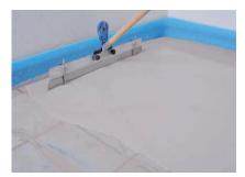
Draw off the fluid load-bearing layer to 9 mm using a pin leveller.
